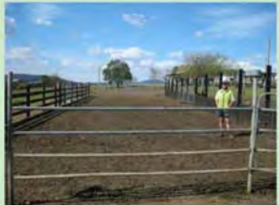
Below: The trafficable solids trap has been constructed using a mould developed by the Mid-north Coast Dairy Pasture Council and funded by Subtropical Dairy.
