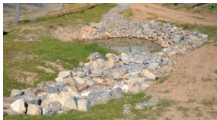
The new sediment basin with rocky outlet
