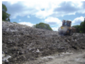
Ripping and reshaping the surface
