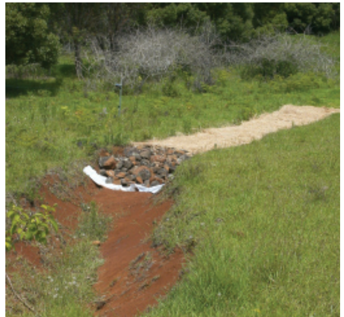
Filling and mulching of the gully
