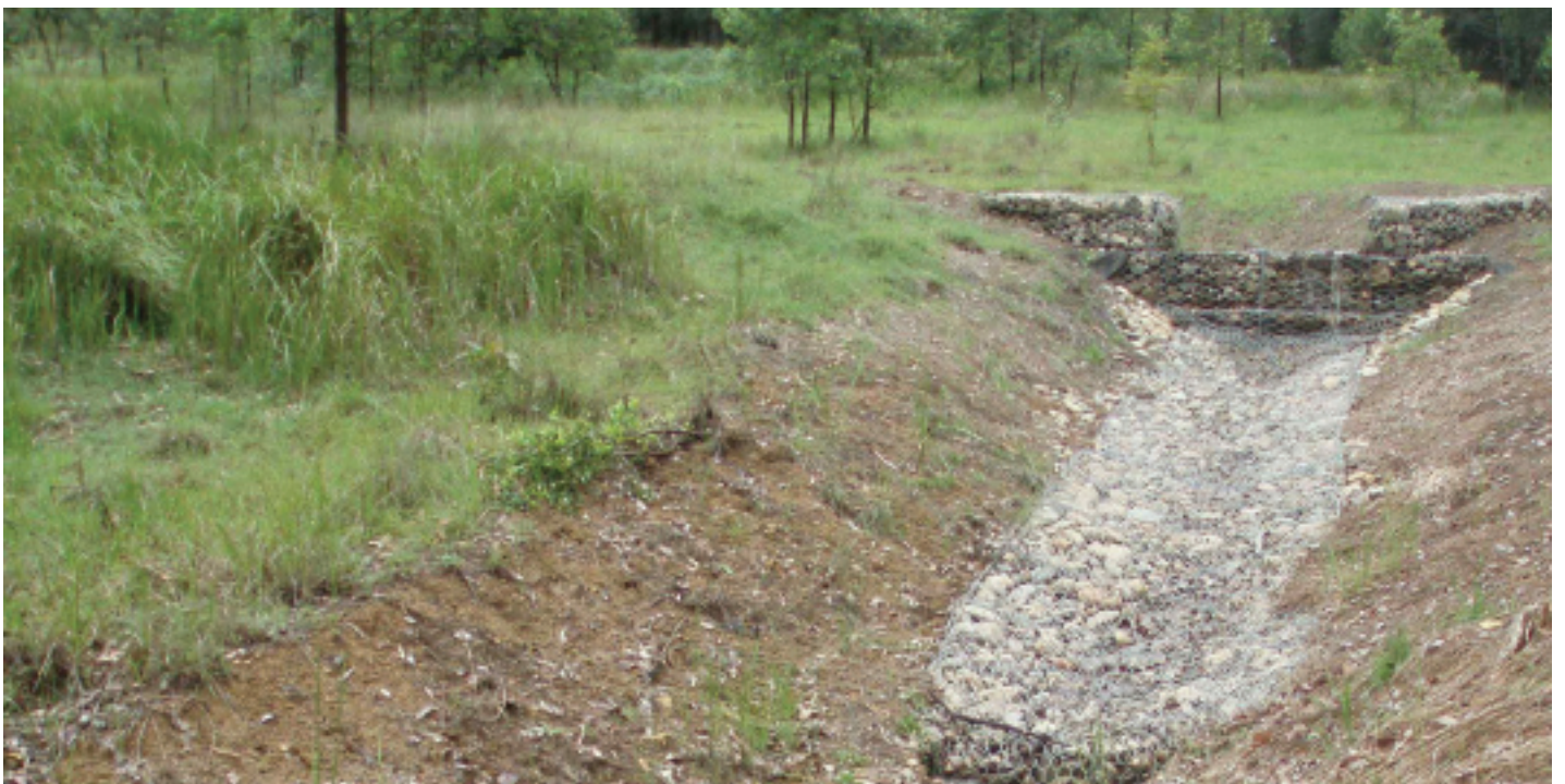
The gabion drop structure that stabilises the dam spillway
