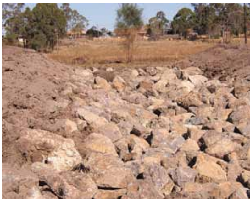
The finished rock chute
