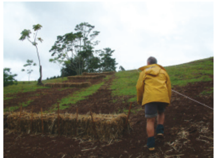
Hay bales slow down water on a steep slope
