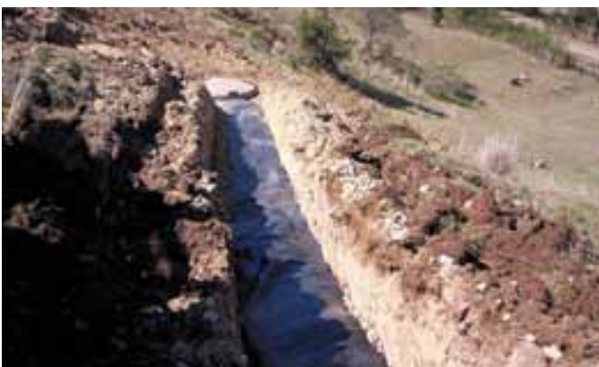
The spring tapper before burial: tapper and geotextile
