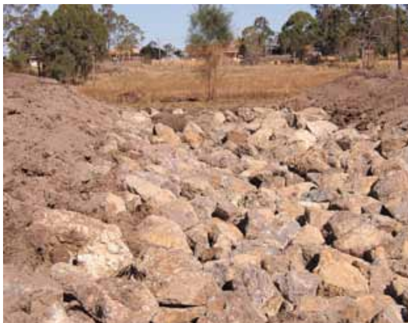
The finished rock chute
