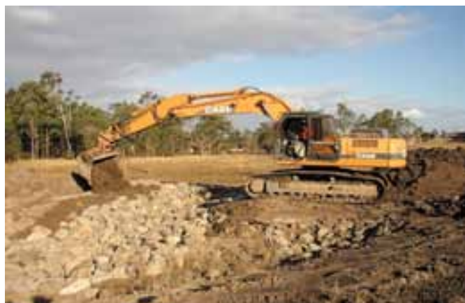
Drop structure in construction
