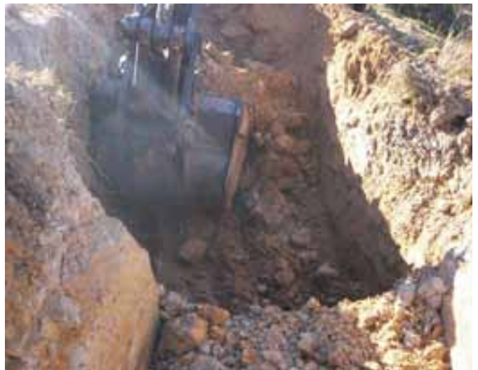
Excavating: spring tapper digging
