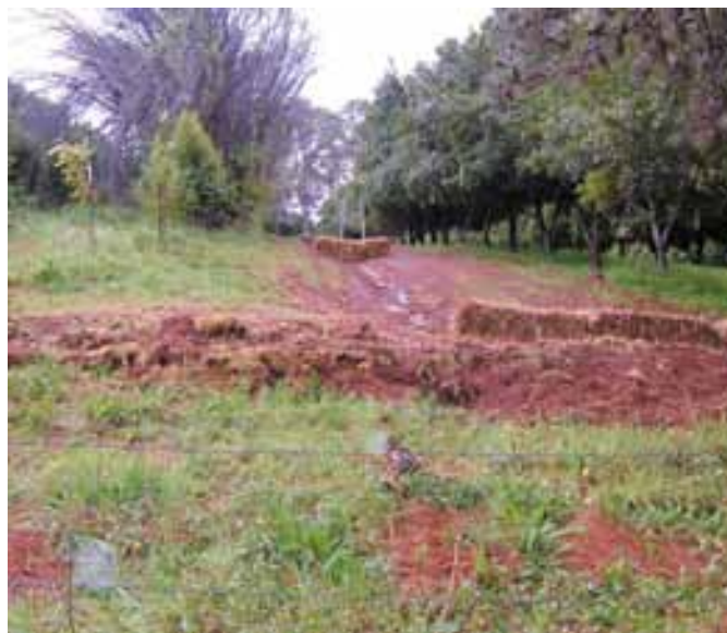
Newly constructed drain with sediment trap
