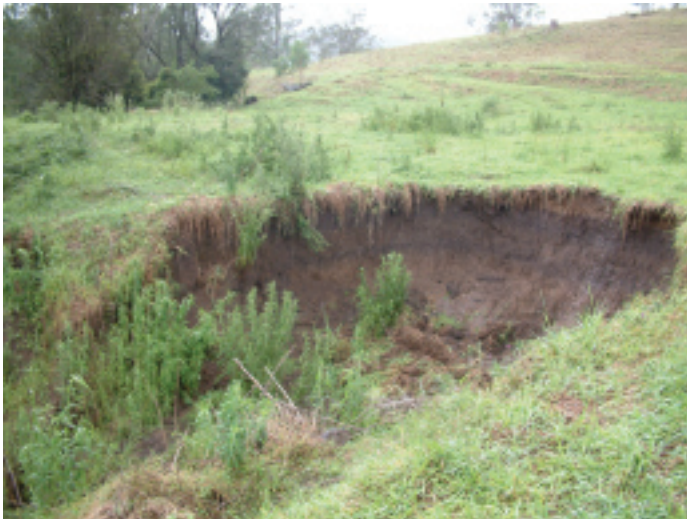
The gully head before works
