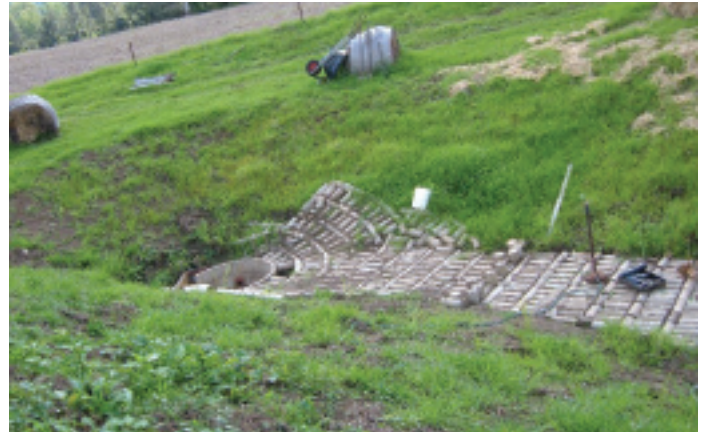
The reshaped gully head area
