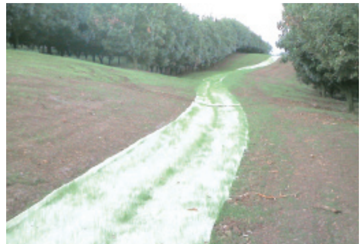
Jute erosion matting laid in the new drain's flowline
