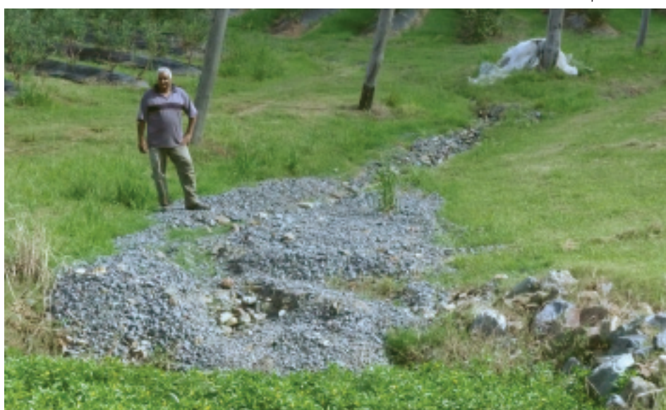
Subsurface drainage improves the central flow line
