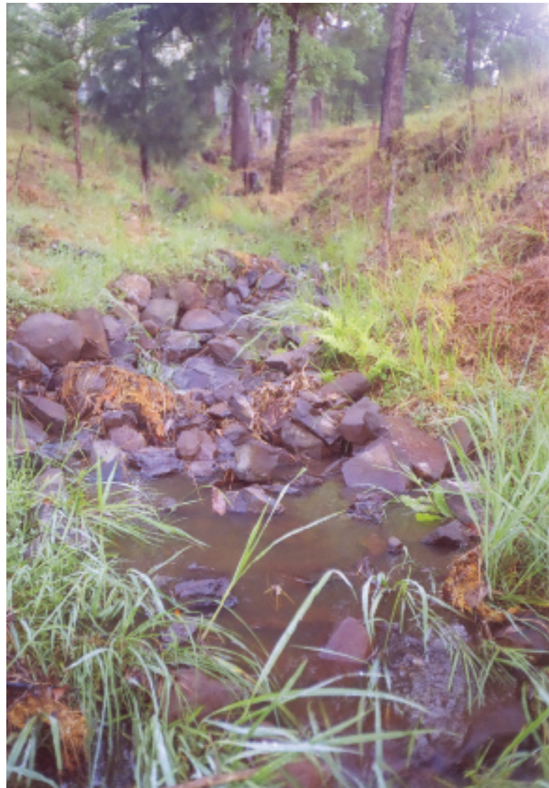
After the flood, rock work has protected the gully
