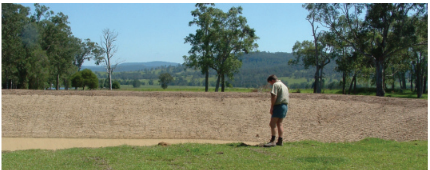
Kevin Coonan inspects the new dam
