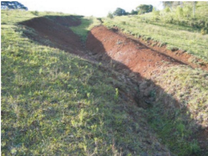
The gully before works
