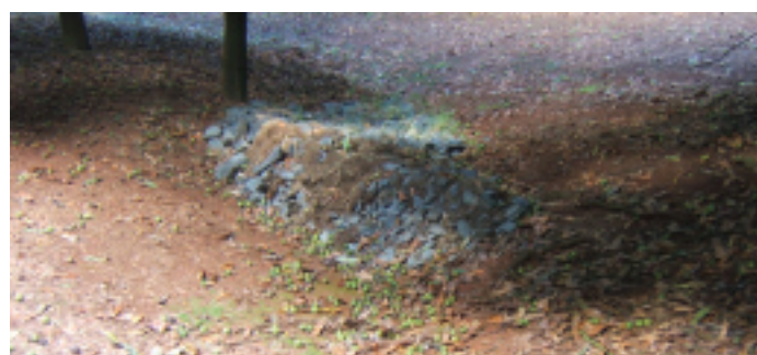
A small check dam protects where water crosses the tree line
