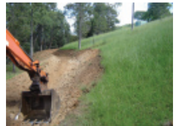
Constructing the diversion drain above the site
